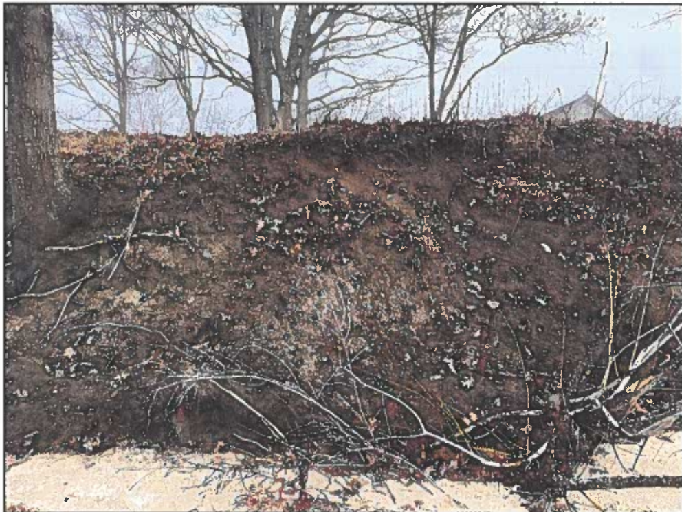
Photograph Four. Additional view of area to be stabilized.
