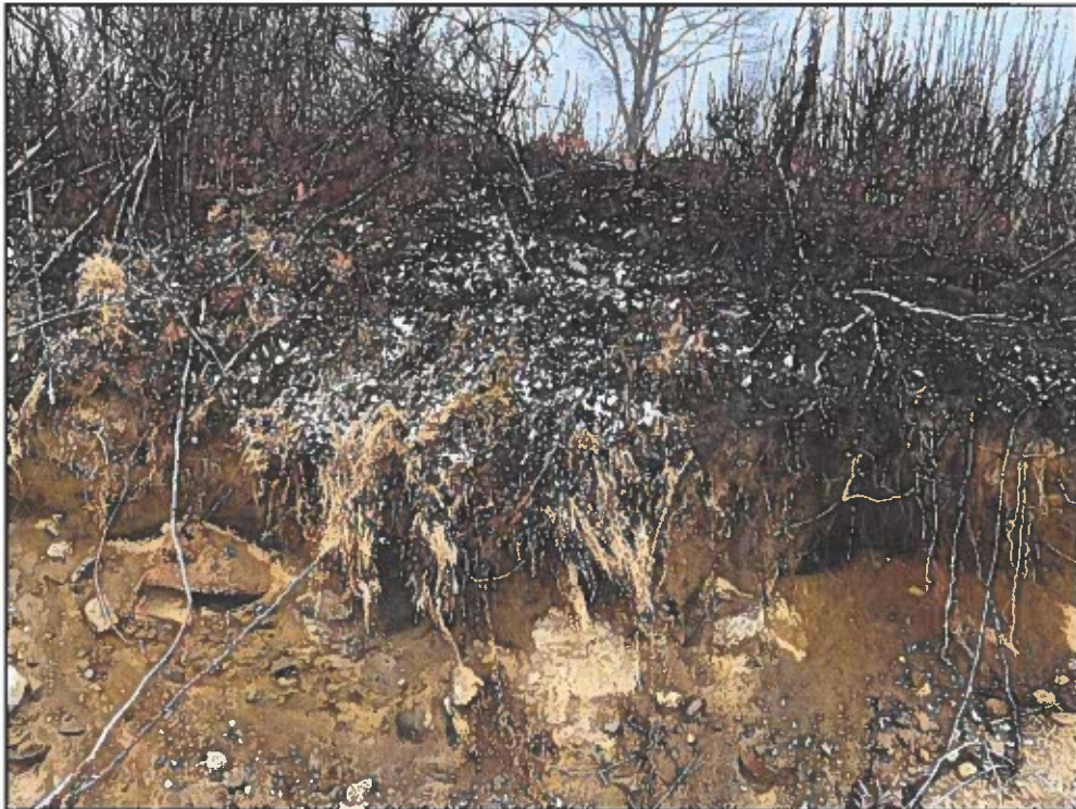
Photograph Six. Additional view of proposed area of stabilization. This location contains a shell midden and will not be graded.
