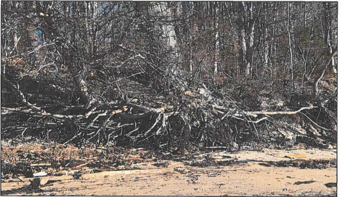
Photograph Three. Additional view of undercut caused by toe scour.
