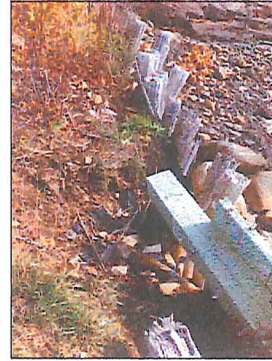
Photo 3 - Erosion behind west end of Bulkhead Section "C" (Bulkhead Section "B" in foreground)
